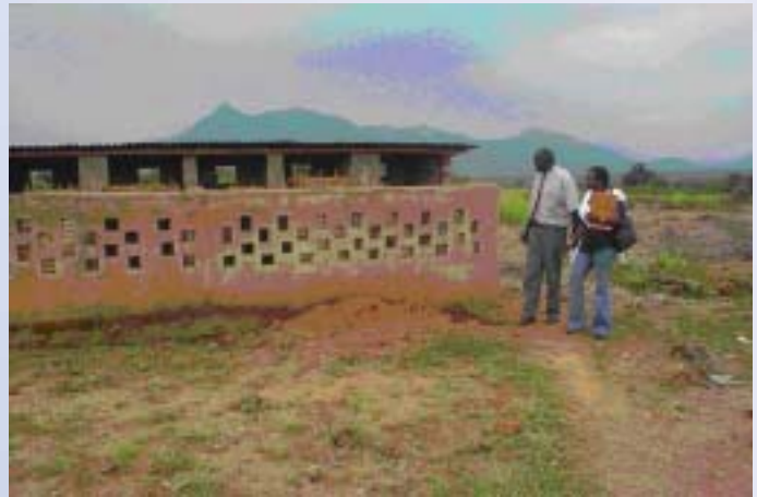
Much needed basics: UNV Perez Abeka (right) and a district official assess the latrine facilities at a school in a return area
